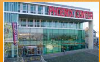
Phoenix Center, Hambourg
